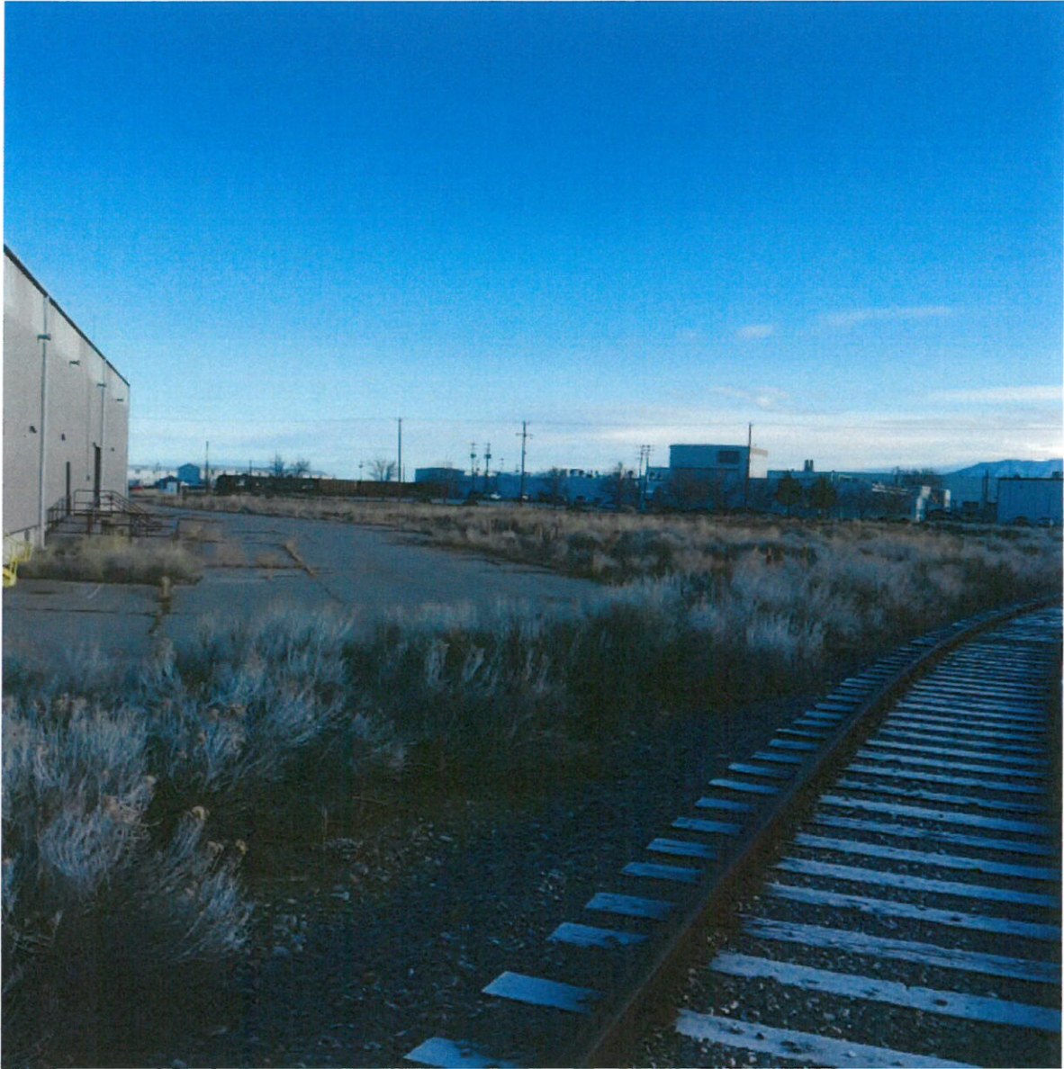
Approximate location for track extension that would serve Building 594. Track would come off of the curve at the middle right of the photograph and lead into the building to the left—building 594.
