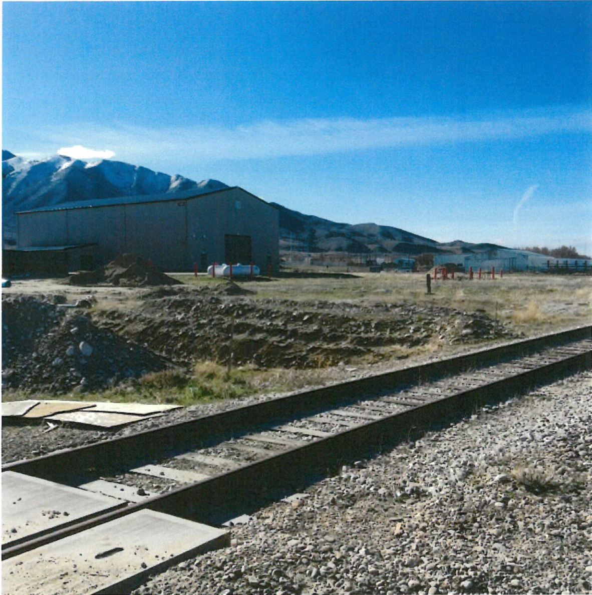
Approximate location for track extension that would serve Building 541. Track would curve from this general area towards the building
