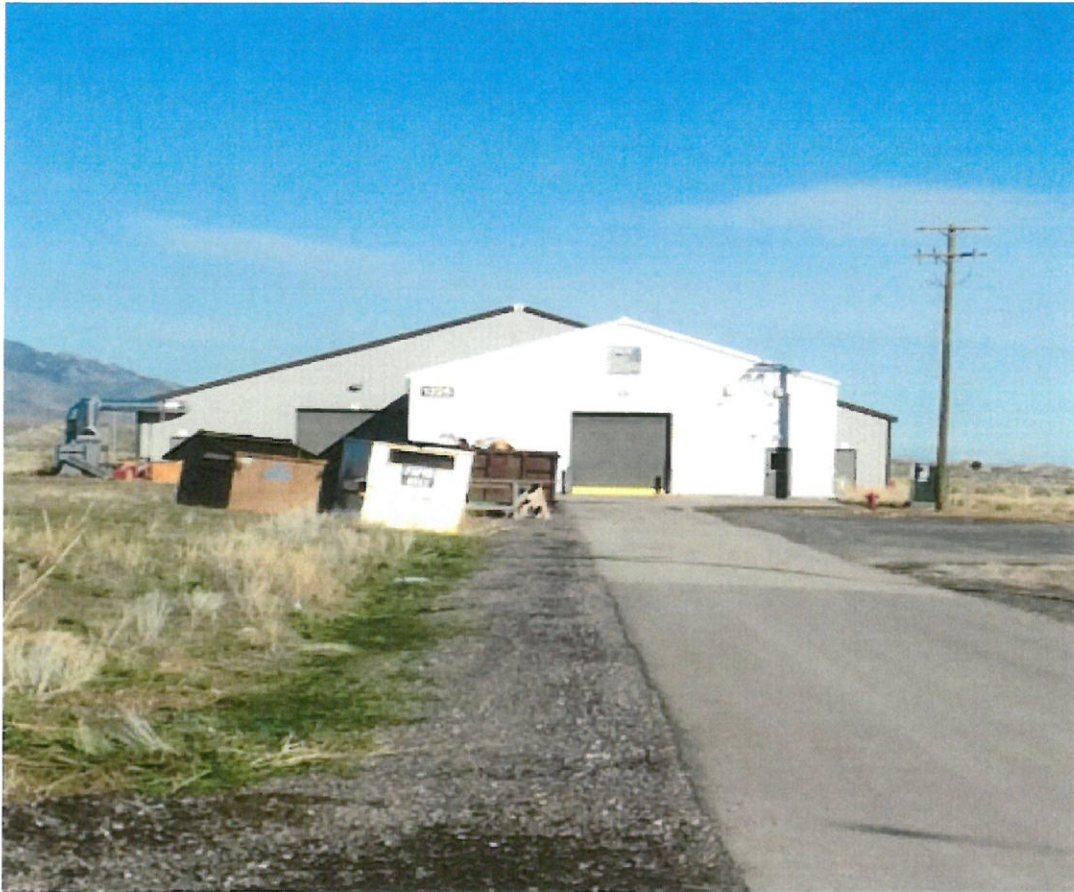
TEAD Building 1225 Constructed in 2000 and is in the ammunition area of TEAD.
